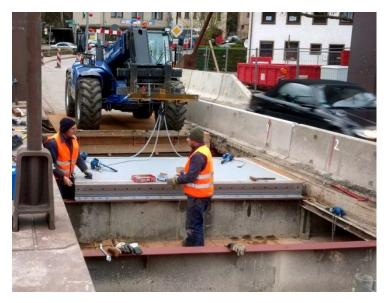
SPS is able to replace orthotropic bridge decks with a new design that has enhanced structural performance. SPS is an isotropic plate with damping and vibration insulation characteristics that also reduces traffic noise emission.
