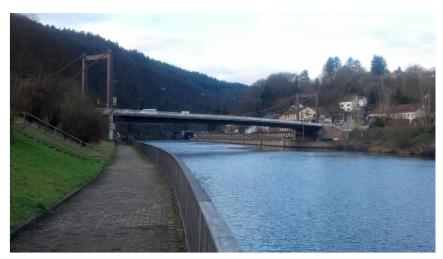
The 1951-vintage suspension bridge crossing the river Saar in Germany at Mettlach needed refurbishing to meet current highway safety standards. The bridge is located in unique "Saarschleife" tourist region and connects the districts of Mettlach and Keuchingen with a double span of 108 m. This is an important traffic connection in the area for which a total closure was not allowed. In the 1950s the
