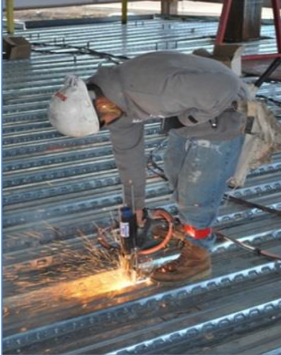
Shear Stud Welded Through Deck
