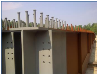
Bridge Girder with 7/8 Shear Studs
