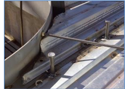
Welded Deformed Bar Anchor
