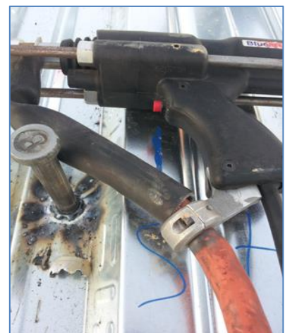
Shear Stud thru deck and Bluearc Stud Gun
