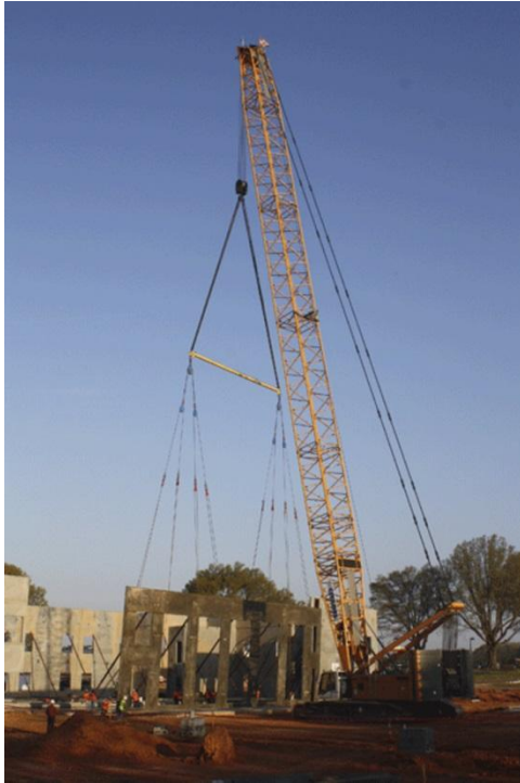
Liebherr LR 1300 crawler crane
